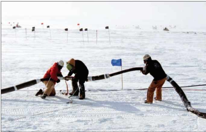
IceCube drillers wrestle the drill hose sections into position. (Image credit: Jim Haugen.)
